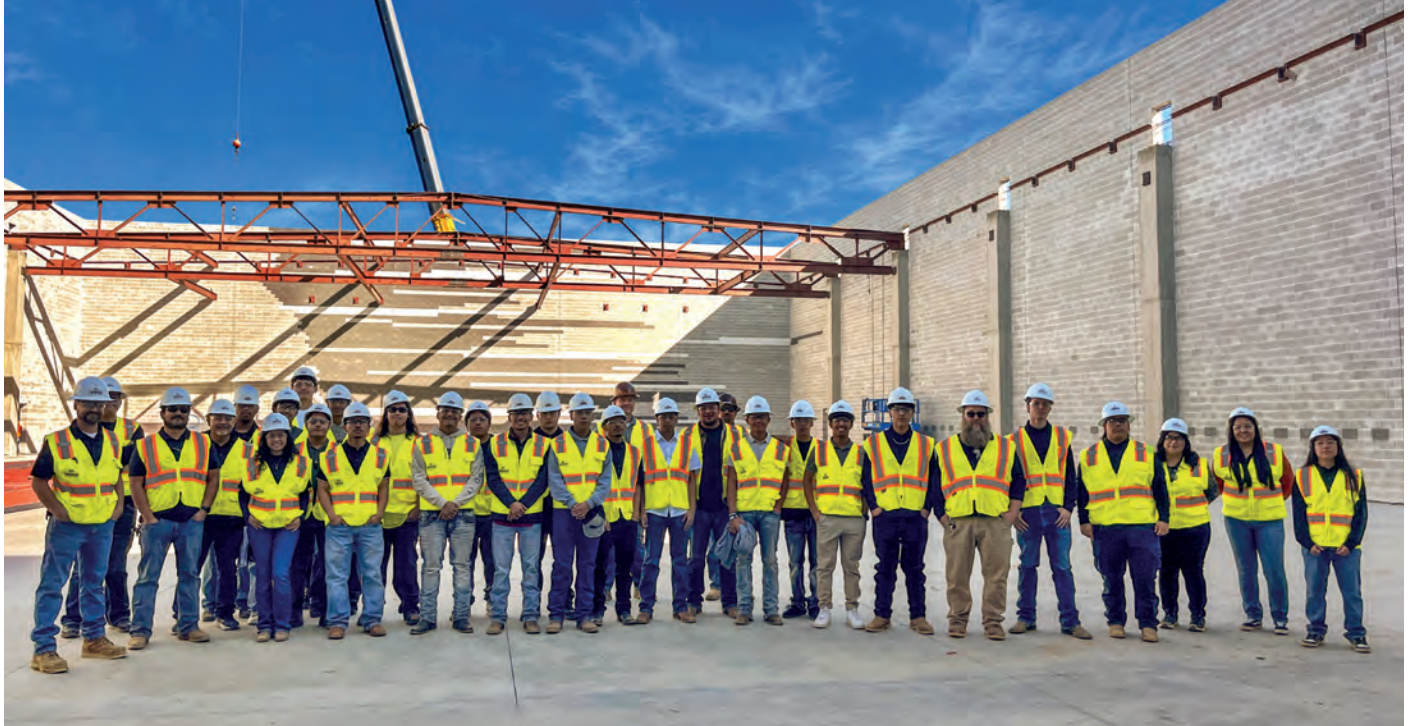
Valley ROP Students tour the gym construction at Phillip V. Sanchez Intermediate School as the trusses were being installed. This is a Harris Construction jobsite constructing both the Phillip V. Sanchez Intermediate School and Clovis South High School located at the Terry P. Bradley Educational Center, Clovis Unified School District.
